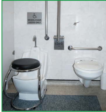
WM COMPACT WITH STOOL WHICH CAN EASILY BE PUSHED ASIDE FOR WHEELCHAIR ACCESS
