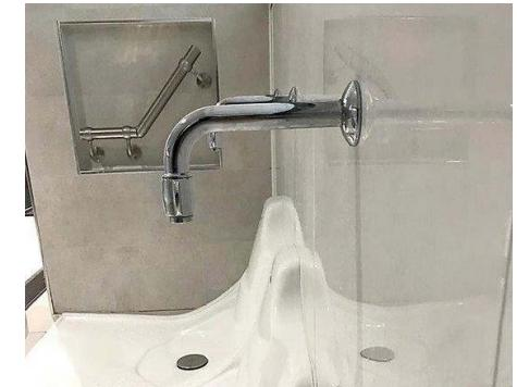
**WuduMate Modular** – The WuduMate Modular can be configured without its stool for standing wudu, and as long as the WuduMate Modular is fitted flush with the floor, wheelchairs will be able to access this. As in this installation, grab bars can be set into the wall to avoid wheelchair hindrance.
