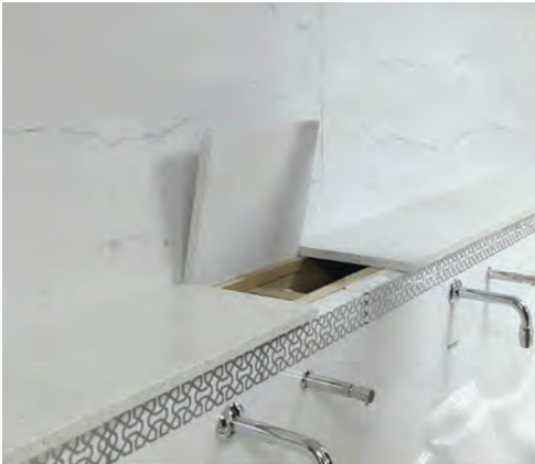
Stud wall showing access to soap reservoirs
