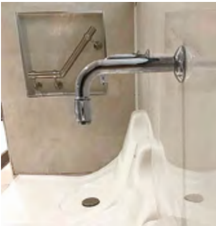
GRAB RAIL FOR DISABLED MODULAR INSET INTO A WALL TO INCREASE SPACE FOR WHEELCHAIR ACCESS
