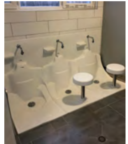
WM MODULAR SHOWING A DISABLED UNIT FOR WHEELCHAIR ACCESS
