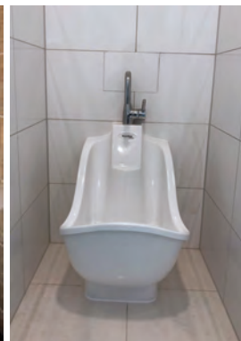
WM COMPACT WITH STOOL REMOVED FOR WHEELCHAIR ACCESS
