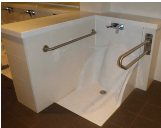
WM MODULAR WITH GRAB BARS AND ROOM FOR WHEELCHAIR ACCESS
