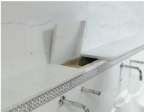
Stud wall showing typical access to soap reservoirs
