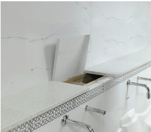
Stud wall showing access to soap reservoirs
